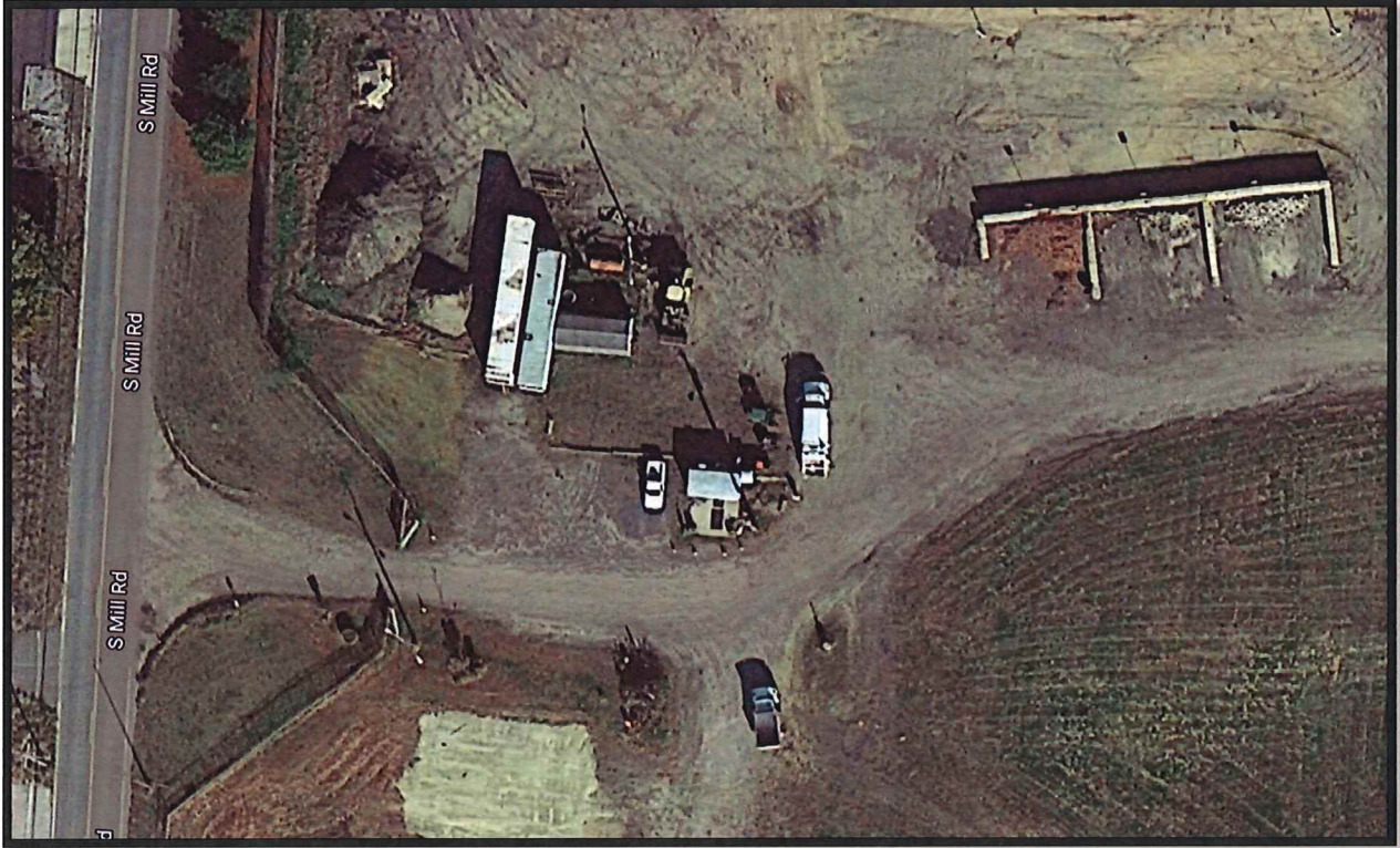
FIGURE 5 Municipal Landfill – Mill Road utility area
