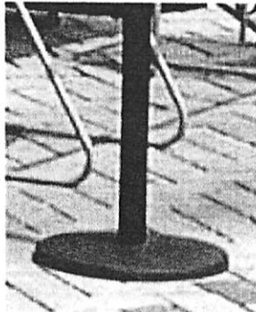
FIGURE 4 Stanchion base must be flat and no more than 1/2" above sidewalk surface
