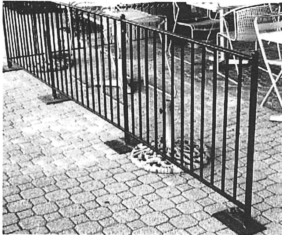
FIGURE 2 Acceptable sectional fencing design
